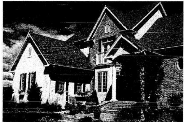
Building Facade Material Example
